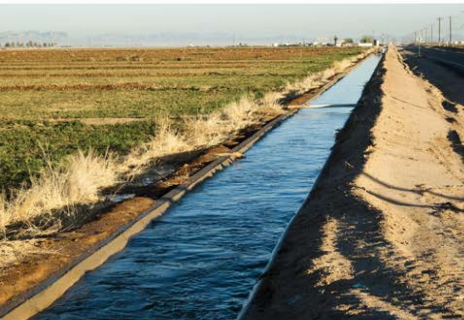
Water Irrigation System
