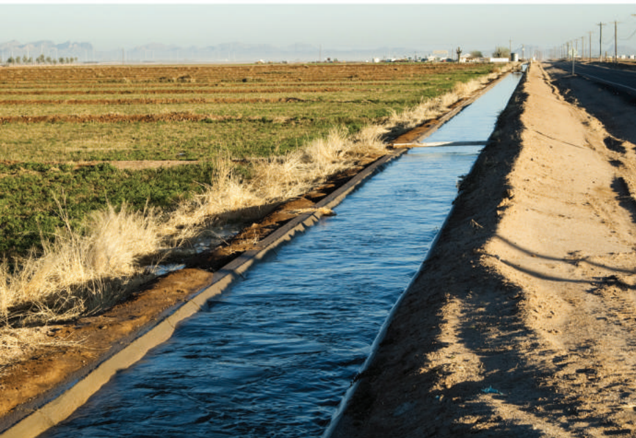
Water Irrigation System
